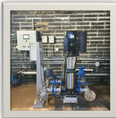
Pump Replacement and pipe upgrade works
