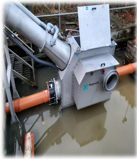
Aughrim Screen Upgrade.
