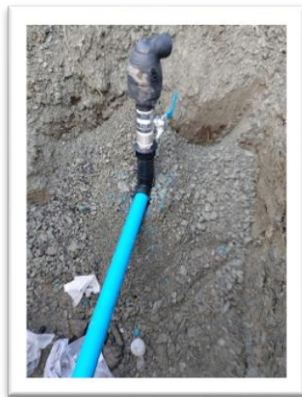
Air Valve replacement, Carnew
