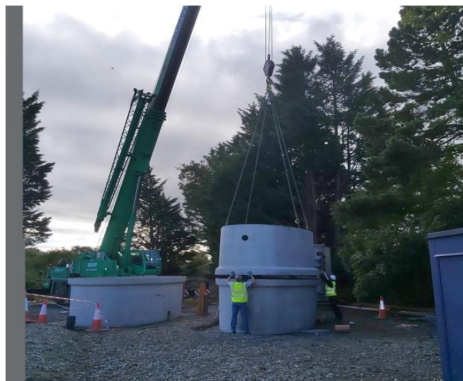
Installation of Settlement Tanks Barndarrig.
