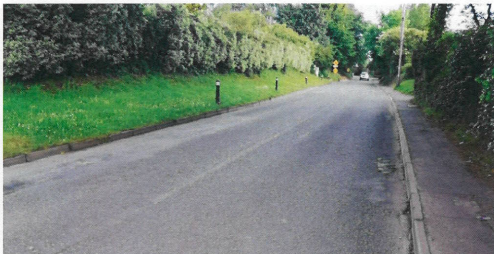
Figure 3.3: Section 1 - Chapel Road - Road Carriageway (Facing North)
