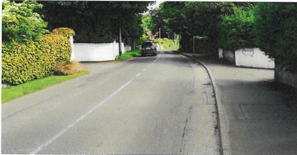
Figure 3.4: Section 2 – Chapel Road – Road Carriageway (Facing North)
