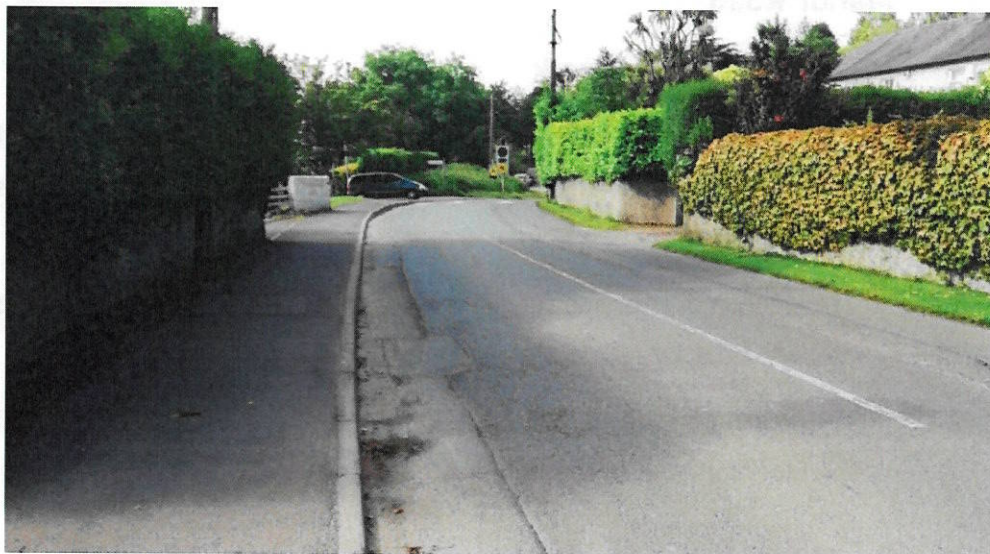
Figure 3.5: Footpath condition along Chapel Road within Section 2 (Facing South)
