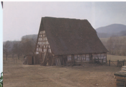
Half-timbered barn in Germany, with a steep roof to throw off snow
