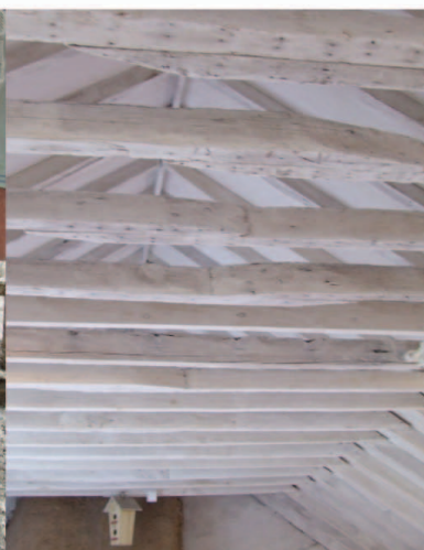
Restored roof in a Wicklow farmhouse conserving original structure with traditionally jointed timbers
