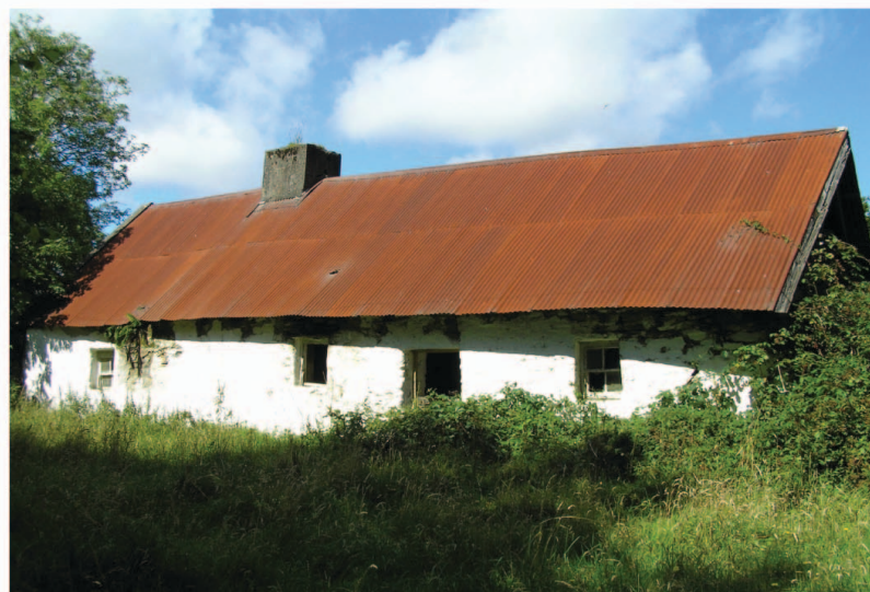
A direct-entry house can be recognized by the position of the chimney away from the door
