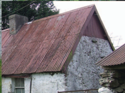
Originally half-hipped roof simplified to a gable
