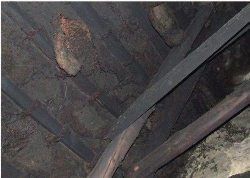
Underside of a thatch roof surviving beneath galvanized iron. Note roof structure of roughly-hewn timber, rope fixings and straw underlayer.
