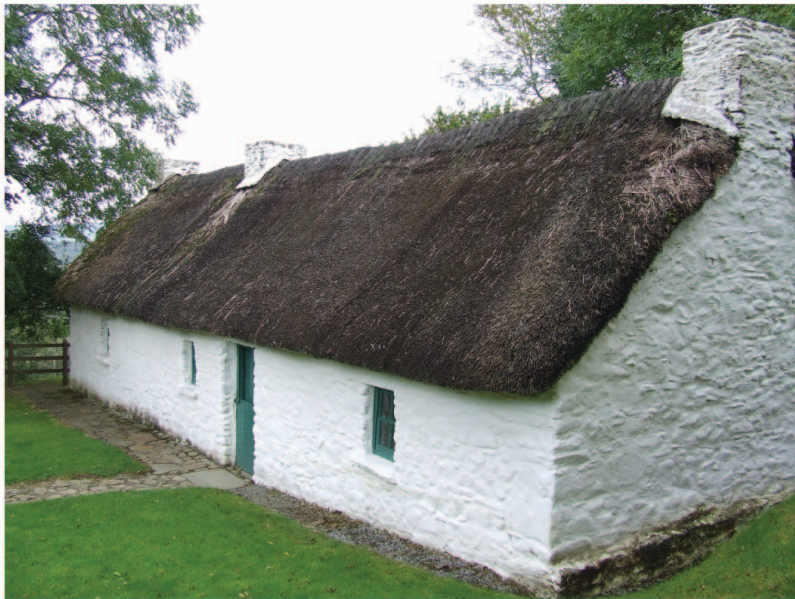
The restored Dwyer-Mc Alistair house with authentic gable-ended thatch roof
