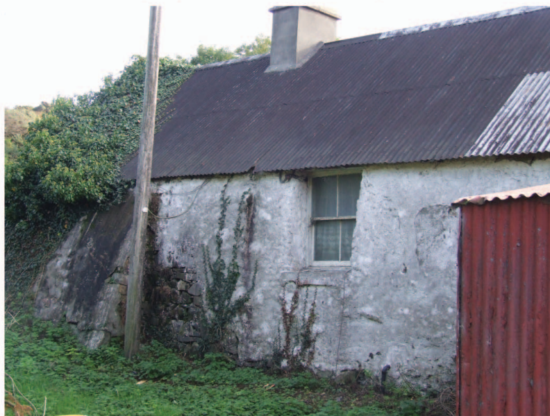
House with battered walls, stone buttress and original lime-washed render
