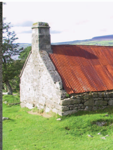
Cut stone chimney near Ballyknockan
