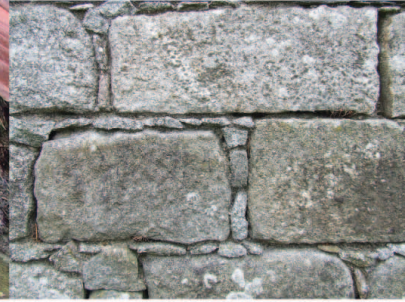
Cut-stone building with distinctive stone “pinnings”
