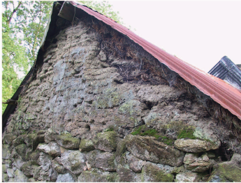
Detail of a stone outbuilding with gable of turf sods. Note the thatch surviving under the iron roof
