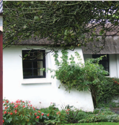
Example of battered mud-wall construction
