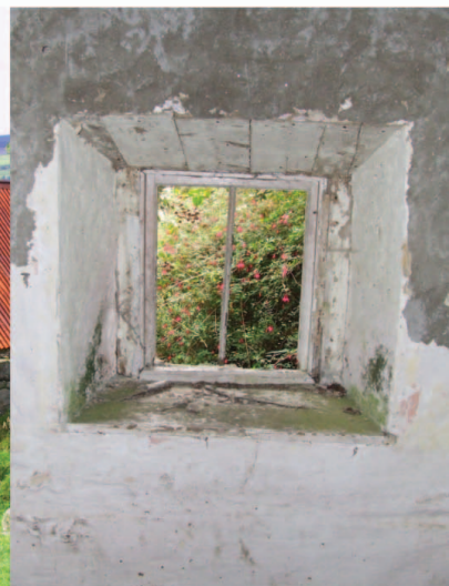
Thick lime-washed walls with splayed window opening
