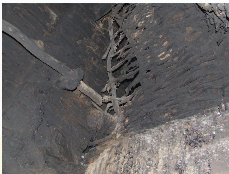
Detail of wicker construction of canopy with rail for hanging pots
