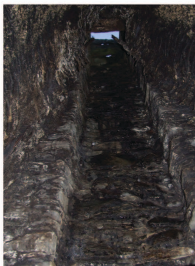
Flue recessed into the stone wall with wicker forming other sides
