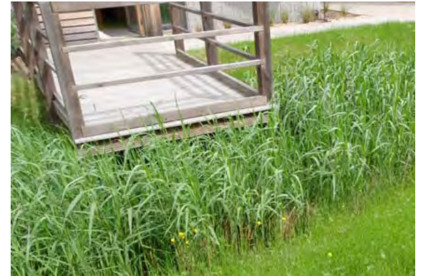
Swale in residential scheme
