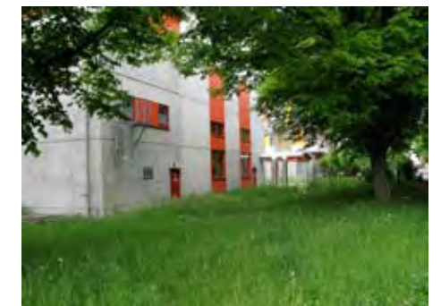
Waste to energy plant in residential area
