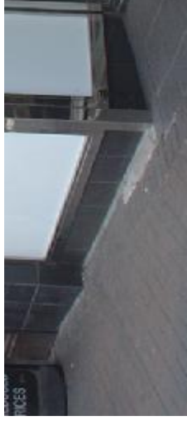
A newer tiled stall riser at Eddie Rockets.
