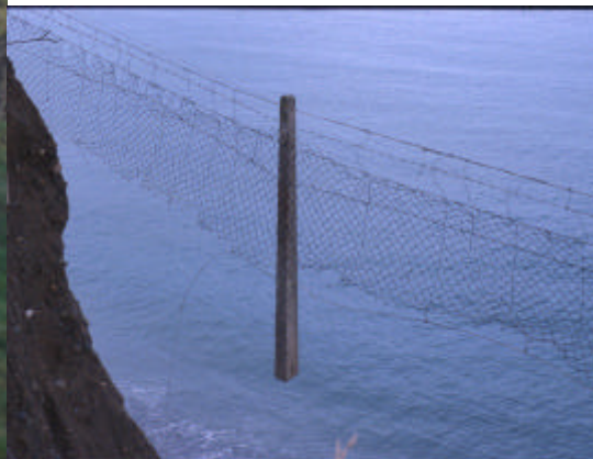
Fence post hanging in mid air due to erosion of sedimentary sea cliffs (Below)
