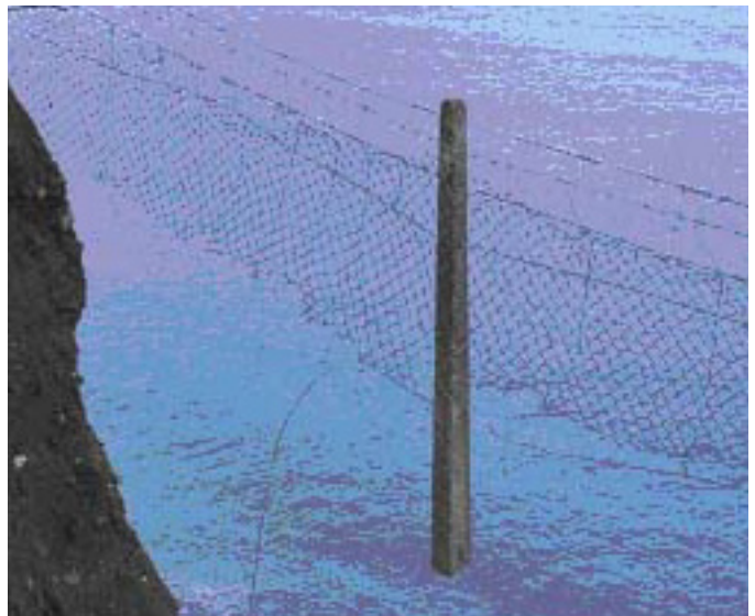
Fence post hanging in mid air due to erosion of sedimentary sea cliffs (Above)
