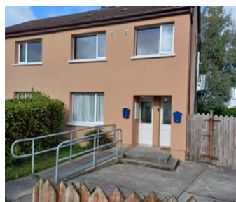
Retrofit Scheme at Monastery Grove. Completed nominated for ICE/LAMA Award
