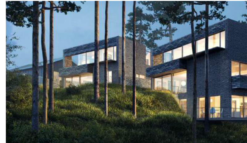
Example of modulated split level massing appropriate for the topography of PLOT B
