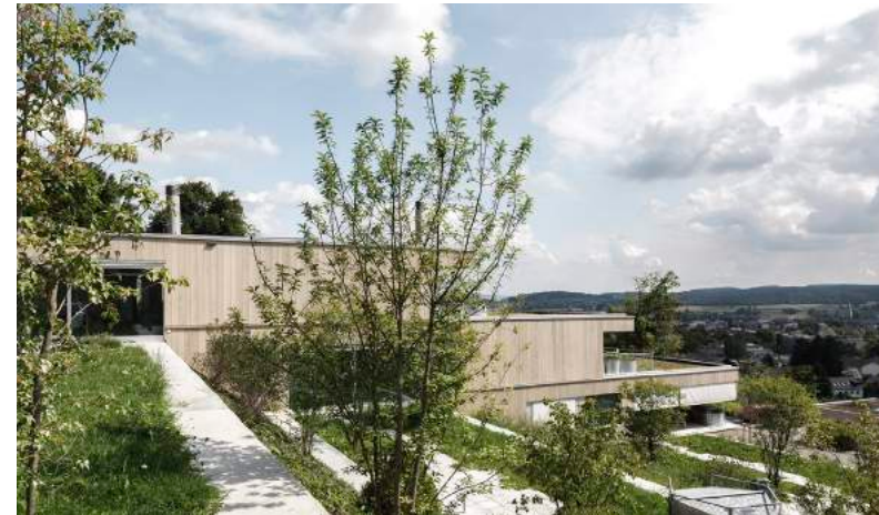
Example of modulated split level housing units appropriate for the topography of PLOT B
