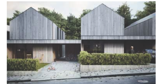
PLOT A Example of modulated housing where the units are required to negotiate a gentle but gradually increasing slope
