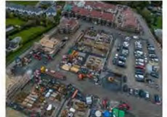
Drone photos taken on 04/12/2022
