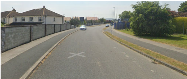
Fig. 15: The quality of the access road toward the Ballycrone Manor residential scheme with footpaths and cycle lanes on both sides (Source: Google Streetview)
