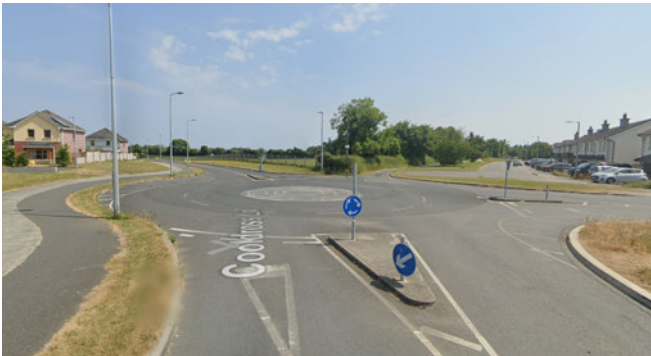
Fig. 14: The quality of the Cooldross Lane/Holywell Avenue roundabout with footpaths and cycle lanes on both sides (Source: Google Streetview)
