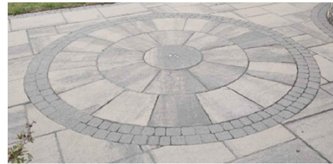
Stage demarcation with flagging + paviours
