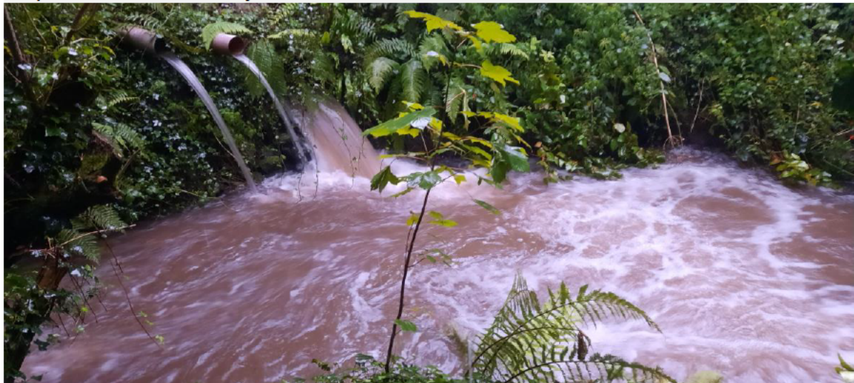
Outfall for surface water into the Marlton Stream on a rainy day
