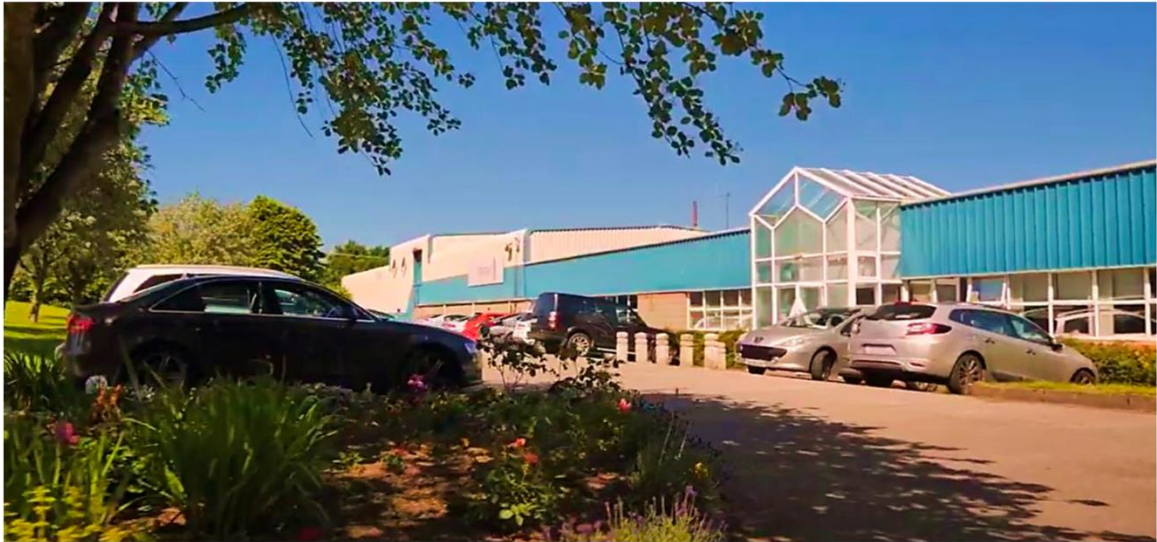
Fig. 08: View D - Existing Building
