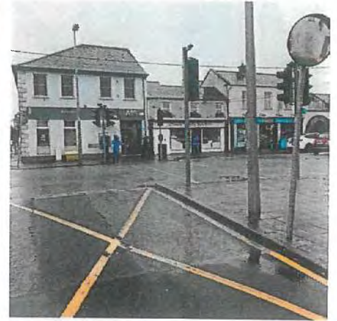
Narrow pedestrian crossing along Main Street
