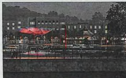
Cobh waterfront public realm improvements by night
