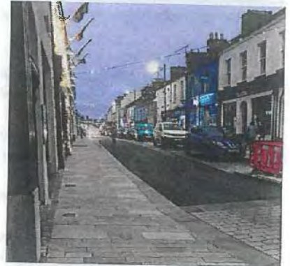
Streetscape improvements and traffic regulations as part of a hand in hand strategy in Carrick-on-Shannon
