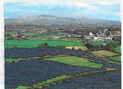
Dale Farm, example of Community Solar Farm
