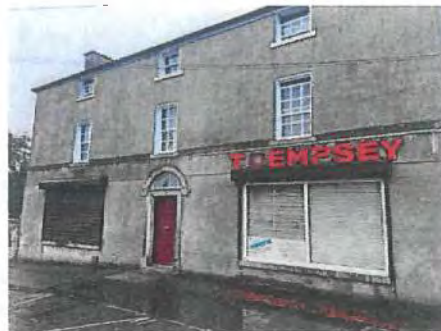
Dempsey's is considered a Building of Special Importance by the Blessington ACA, featuring a timber panelled central door with fanlight over a moulded surround.
