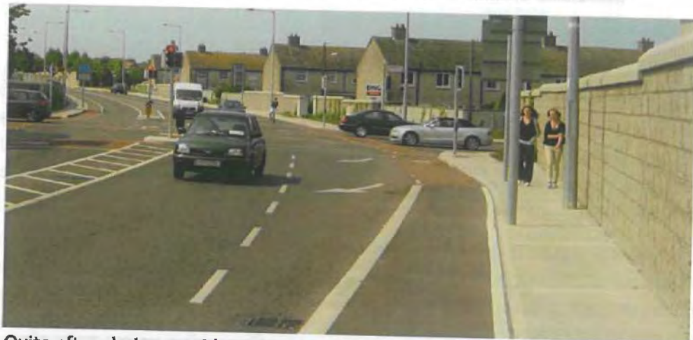
Figure 83 An example of street design where pedestrians are marginalised (DMURS)
