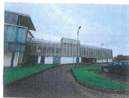
The multi-storey car park within the Town Centre development is an existing but under-used resource within the town. Exploring the potential for reopening the upper floors would ease on-street congestion.
