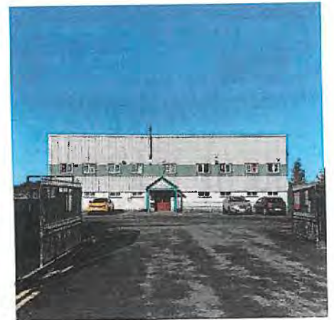
St. Kevin's Community Centre, Main Street
