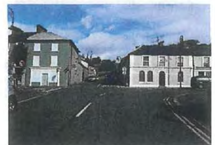
Refurbished residential accommodation in Cappoquin
