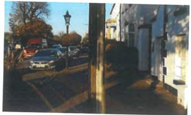
Figure 38 Example of poorly placed service poles
