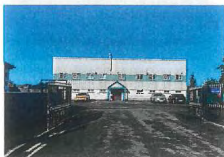
St Kevin's Community Centre, Main Street
