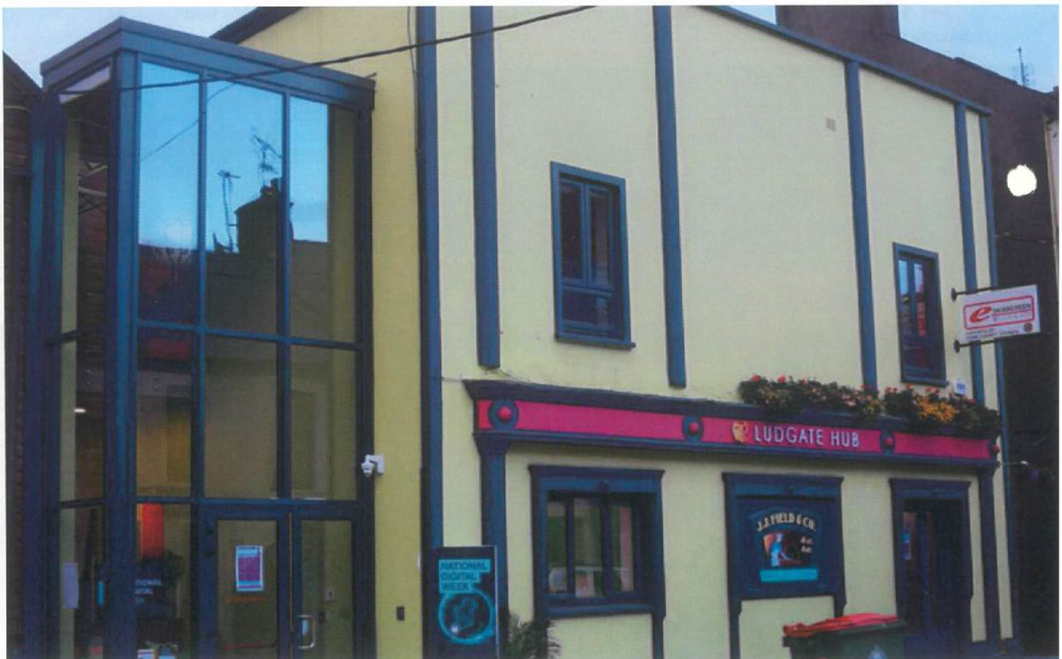
Figure 69 The Ludgate Hub in Skibbereen is a successful digital co-working space that reused a vacant building
