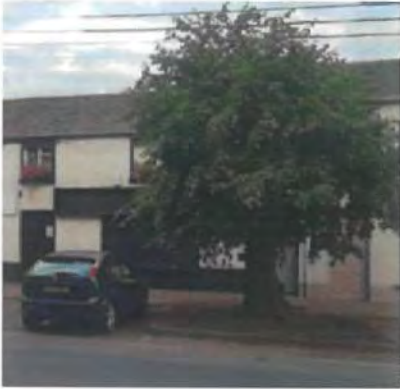
Figure 47 Overhead cabling has led to tree crowning
