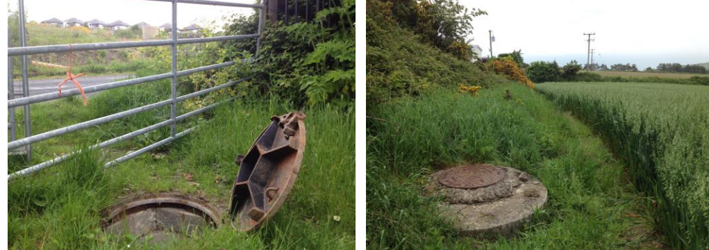
Figs. 3 & 4: Photos of existing foul manholes on the land.
