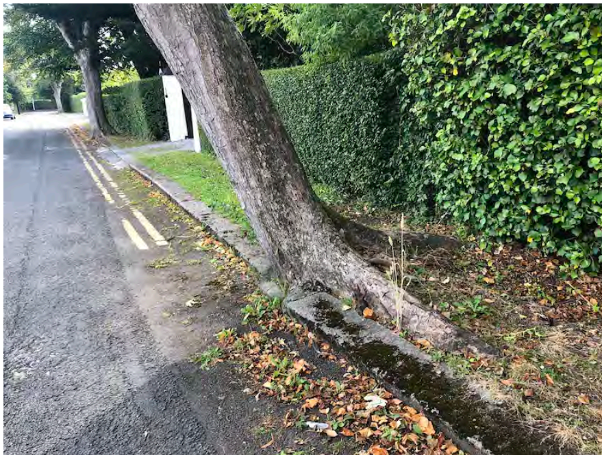
Fig. 33: View of tree causing damage to cast concrete kerb while being at risk of falling.
