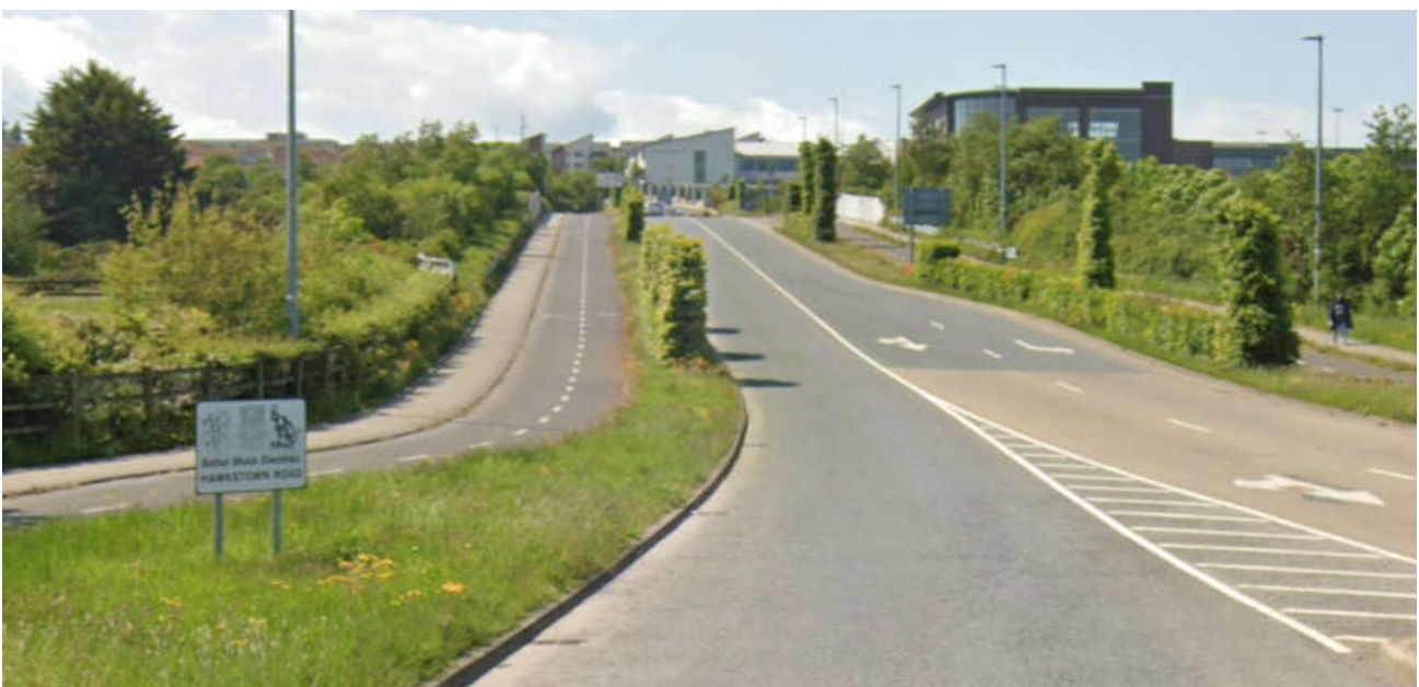
Photograph 3: The site is split by the recently completed Wicklow Town Relief Road.
