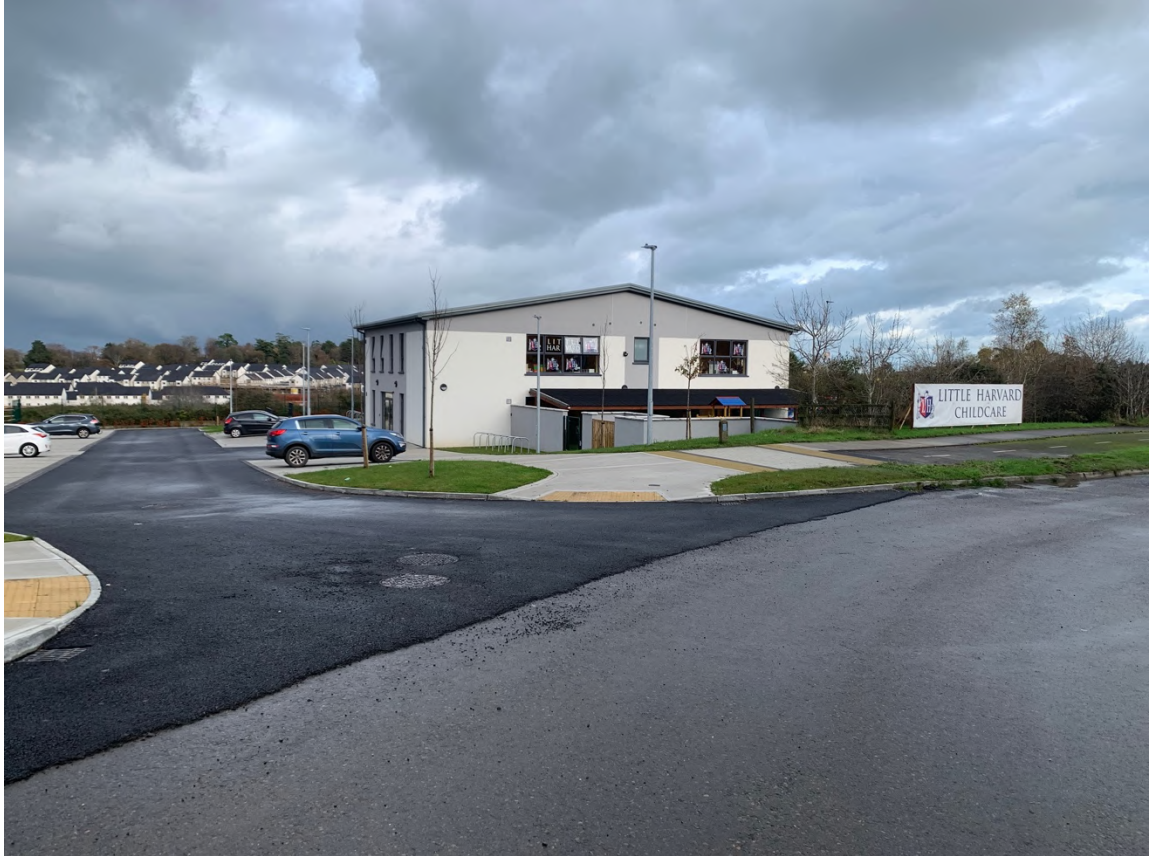
Figure 5 – Operational Creche Facility at Broomhill.
