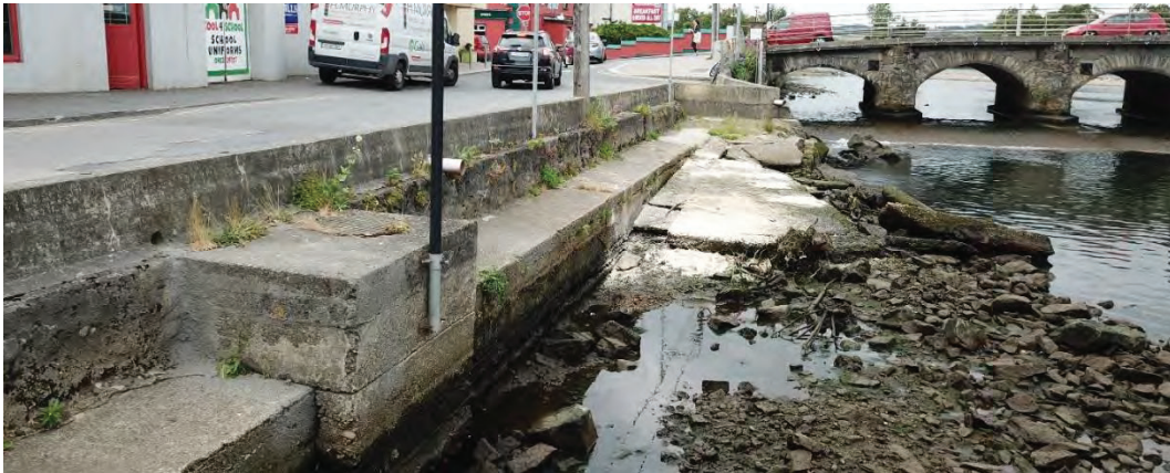
Figure 12.7: Sewer housing and inspection chambers on river side of quay wall.
