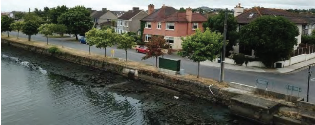
Figure 12.8: Exposed stone quay wall with stone cappings downstream of South Green
